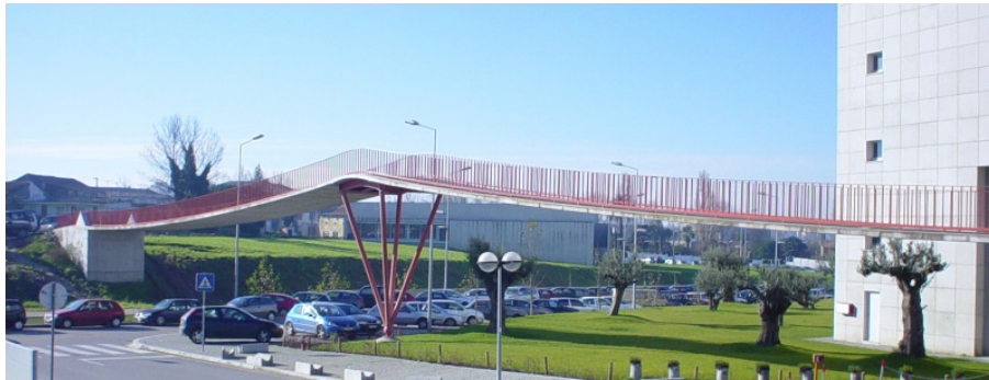
Fig. 24. Stress-ribbon footbridge at FEUP Campus.
