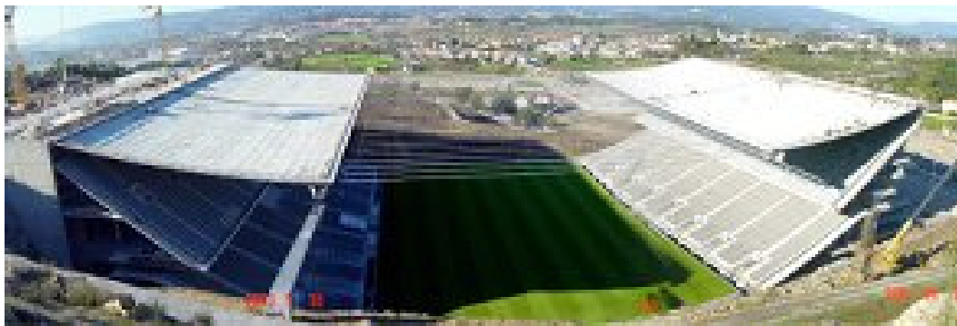
Fig. 18. Braga stadium cable roof.
