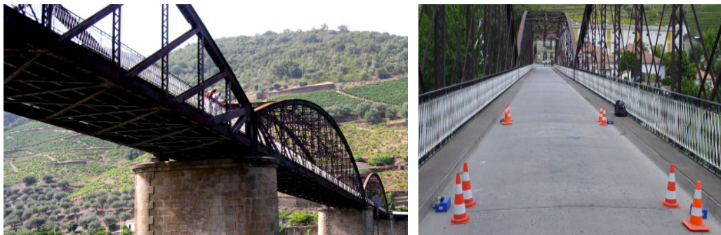
Fig. 23. Views of Pinhão Bridge, over Douro River.
