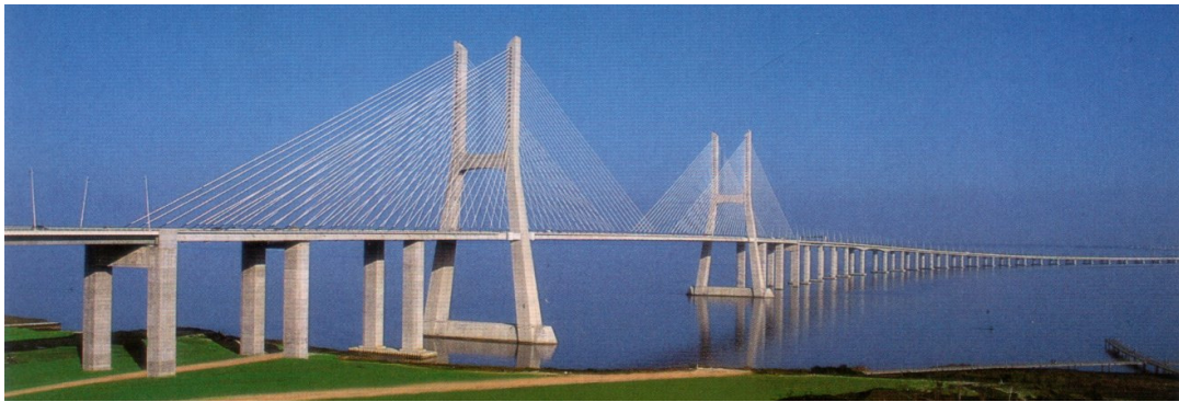
Fig. 14. View of Vasco da Gama Bridge.
